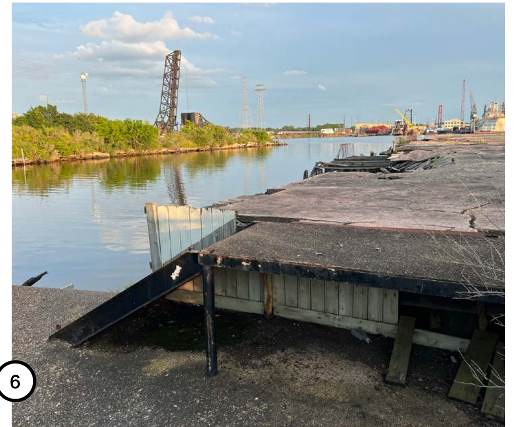
6 Warehouse pier condition
