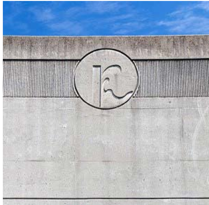
Richmond Flood Wall.
