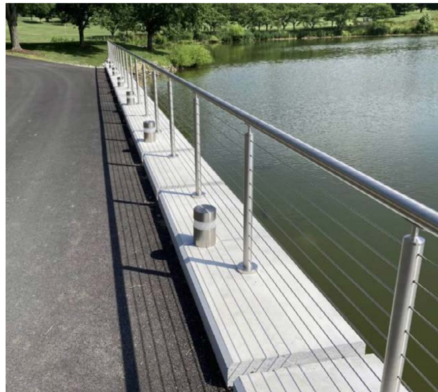
Cable Railing on Top of Wall
