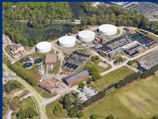
Moore's Bridges Water Treatment Plant
